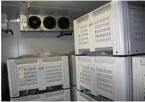
Figure 10. Room Cooling
