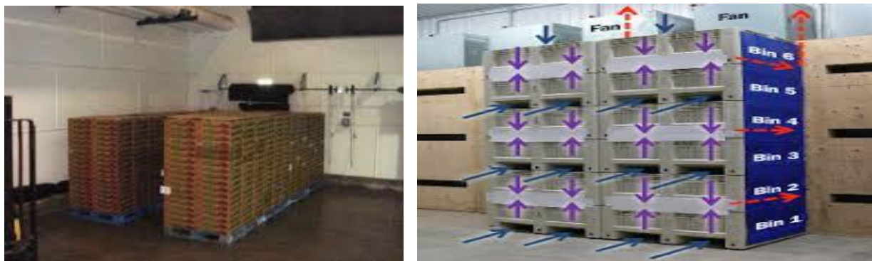
Figure 11. Forced air cooling
