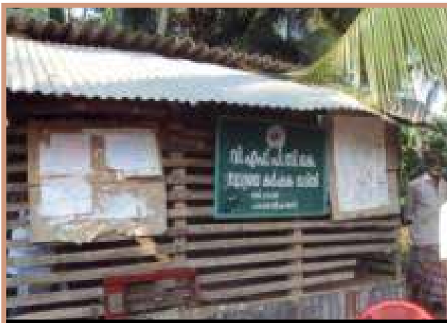
Fig 72: Cluster Mini Mandi in Thiruvananthapuram (VFPCCK managed)
